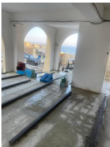
Figure 4: Area of overflow
