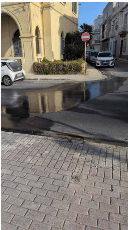
Figure 1: Overflow into the street
