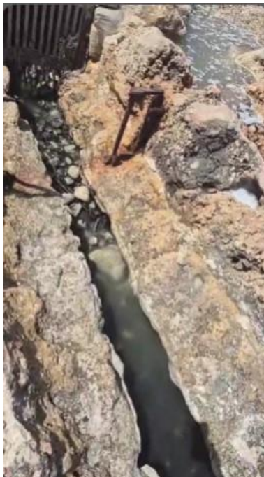
Figure 3: foul water percolation
