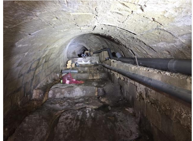
Figure 4: change of main sewer inside the tunnel
