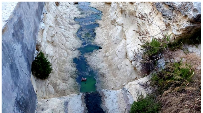
Figure 2: Green Dye carried out from main sewer
