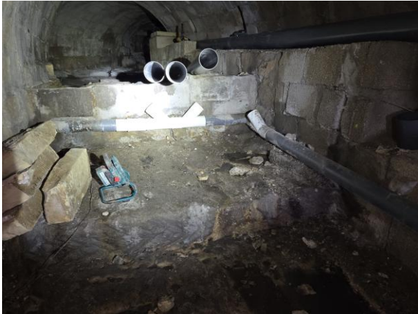
Figure 3: Change of main sewer inside the tunnel
