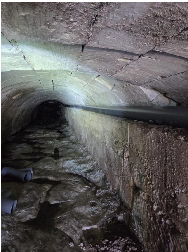
Figure 5: change of main sewer inside the tunnel
