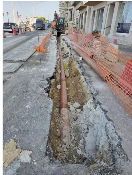
Figure 7: main sewer replacement
