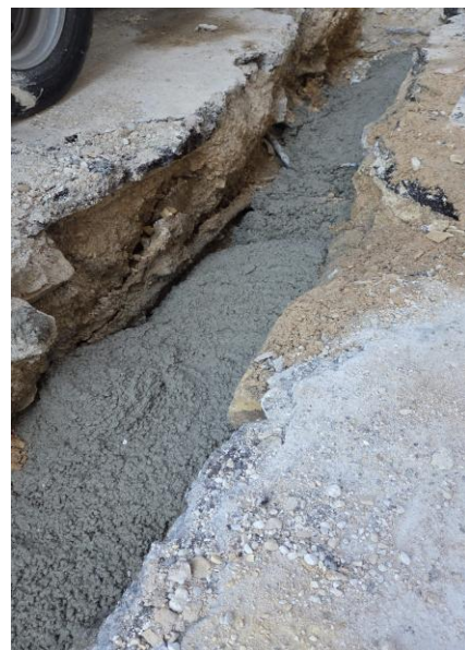
Figure 9: works completed and sealed
