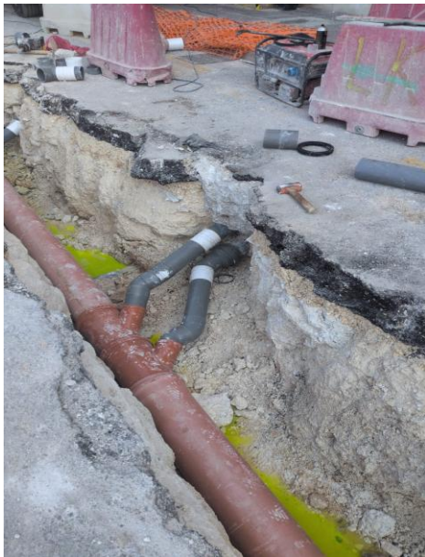
Figure 6: colour test to check works
