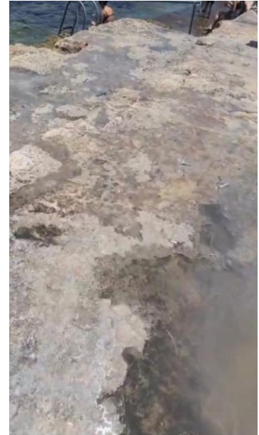
Figure 3: Overflow going into the sea
